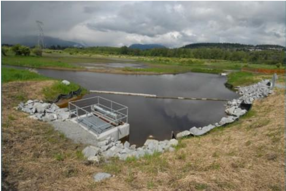
Figure 3: Exit point, or upstream end, of self-regulating tidegate. Photo by Zach Sherker
