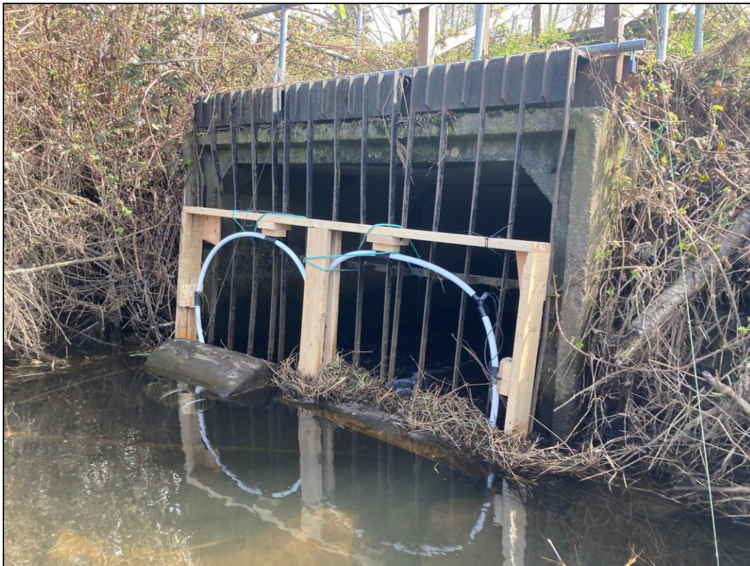
Figure 8: Antenna installation at Sheep Paddocks floodgate (control) site. Photo by Zach Sherker
