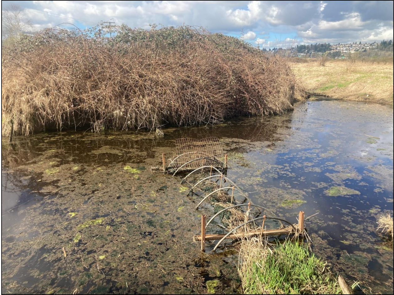
Figure 4: Top-mounted floodgate. Photo by Zach Sherker
