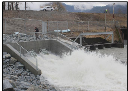
Figure 1 Hatzic Lake Pump Station
